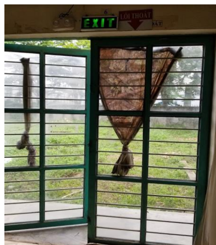
Figure 3: Exit Door ‘Pinned’ Partially Open
