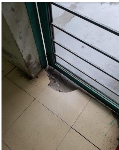
Figures 4 – 5: Broken Flooring at Exit Doorway
