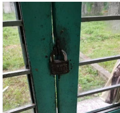
Figure 2: Locked Exit Door
