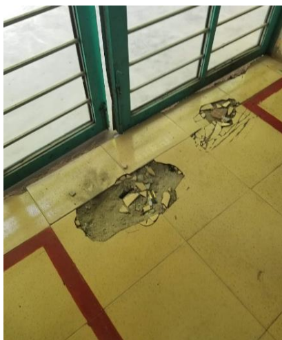
Figures 4 – 5: Broken Flooring at Exit Doorway
