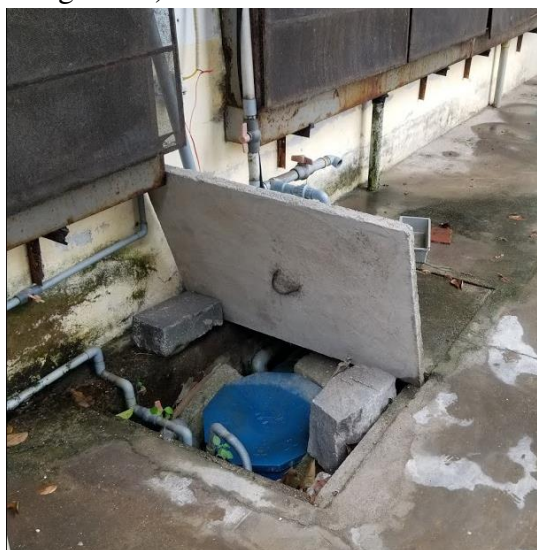
Figure 36: Heavy Concrete Cover for Evaporative Cooling System Sump
