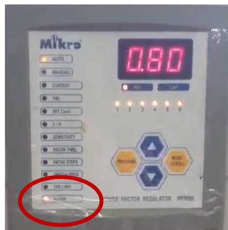
Figure 28: Electrical Panel with “ALARM” Warning Lit
