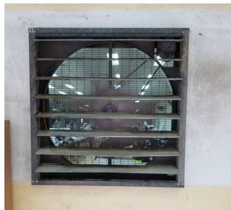
Figure 16: Unguarded Fan Blades inside Dampers
