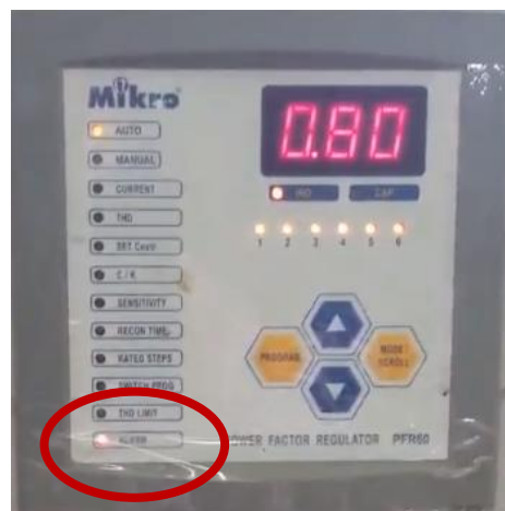
Figure 28: Electrical Panel with "ALARM" Warning Lit
