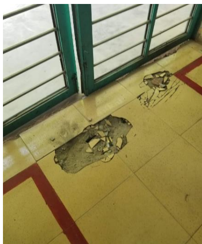
Figures 4 – 5: Broken Flooring at Exit Doorway
