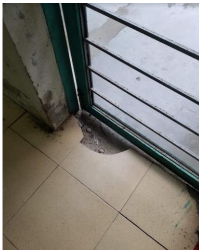
Figures 4 – 5: Broken Flooring at Exit Doorway
