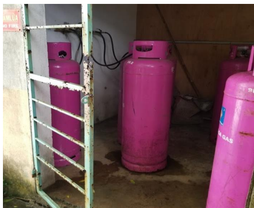
Figure 9: Unsecured Gas Cylinders
