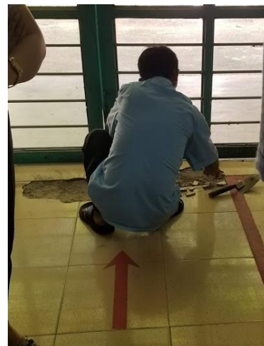
Figure 6: Employee Repairing Broken Flooring
