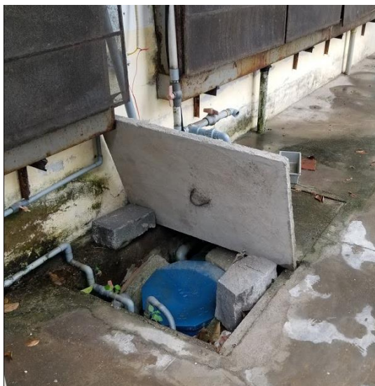
Figure 36: Heavy Concrete Cover for Evaporative Cooling System Sump
