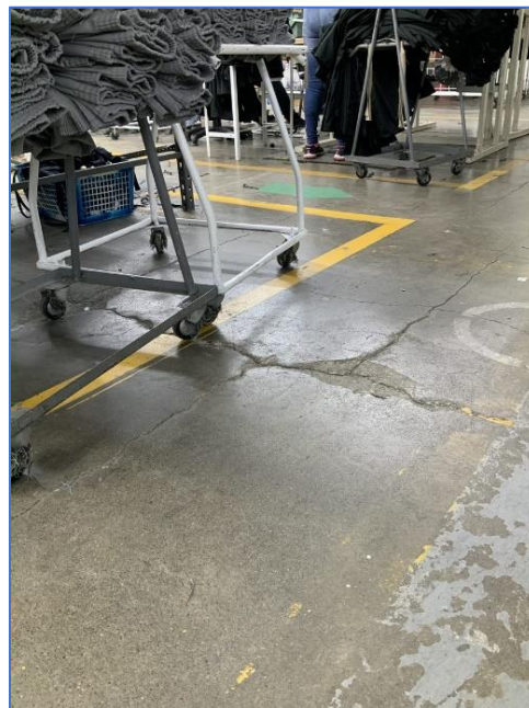
Figure 15: Cracked floor surfaces
