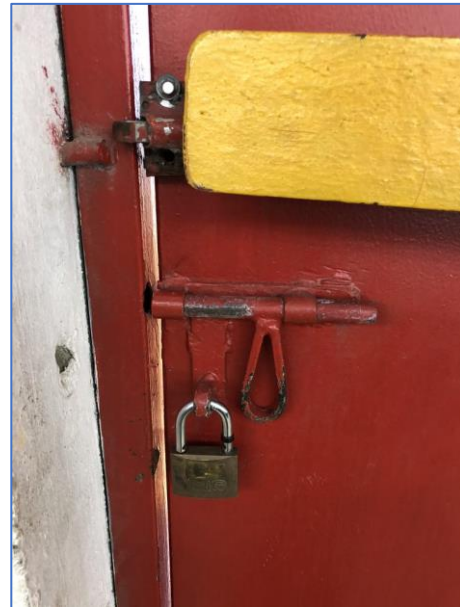
Figure 3: Emergency exit doors equipped with hasps and locks
