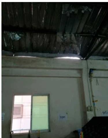
Figure 9: Leaking Roof in Eating Area at Honeys 1
