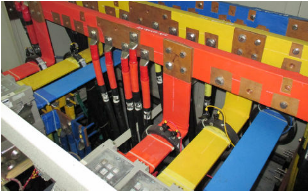
Electrical Bus Bar in LT Panel at an Accord-covered factory, after remediation. Proper maintenance ensures that all elements are kept free of dust and dirt, which prevents malfunctioning and electrical short circuits.
