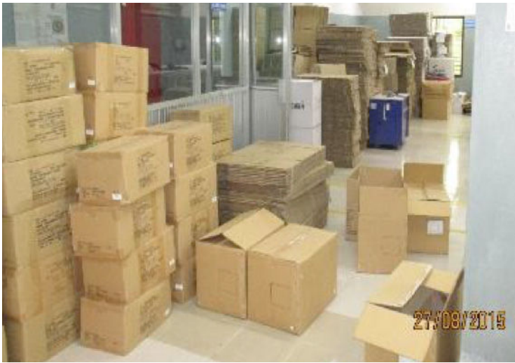
Storage blocking the means of egress, which prevents a safe evacuation of the factory in case of fire or another emergency.
