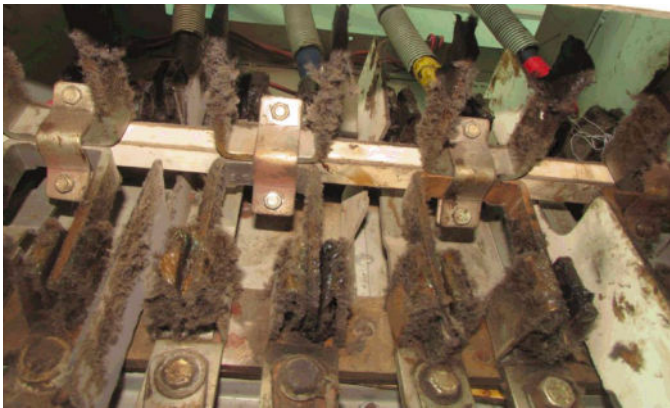
Dust and dirt accumulated on electrical wiring, which can cause sparks and start a fire. This fire hazard was identified at over 60% of the Accord-covered factories.
