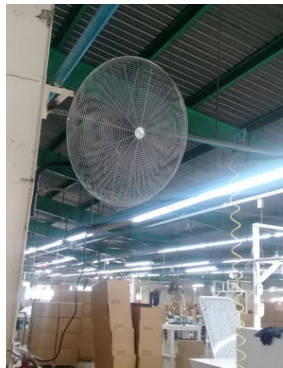
The installation of additional fans helps to provide additional ventilation.
